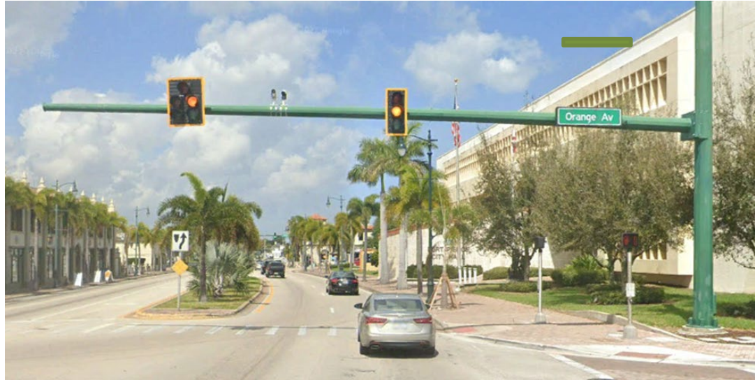
Traffic signal backplate installations for increased visibility of signal lights
